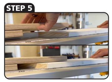
SLIDE CUT END OF CASING UNDER THE DOUBLE STOP TILL LONGEST END TOUCHES THE BOTTOM PIECE.
