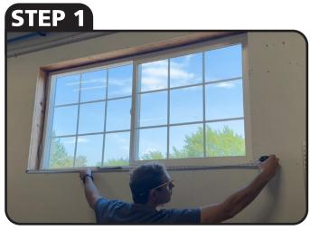
FIND INSIDE MEASUREMENT OF DOOR/WINDOW CASING
